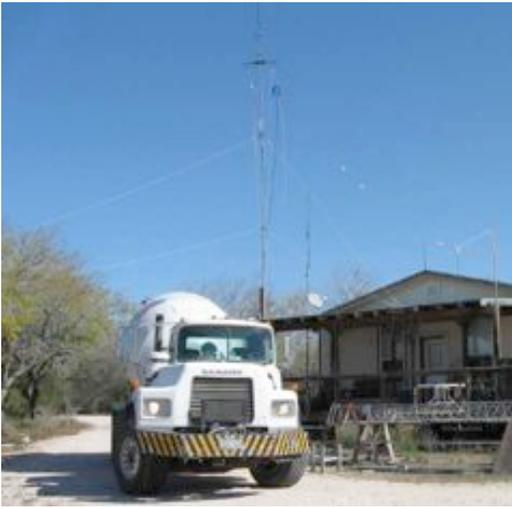
cement truck. They poured a little cement in the bottom. Charles used a cement vibrator to spread it around and checked the level of the base. It was still in line so they poured some more. Charles vibrated the cement and checked the level. This went on for what seemed to be hours until finally the hole was topped off. The wood braces for the tower base were still seeming to be level.
